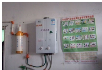
Water heater with desulfurization equipment and shower
