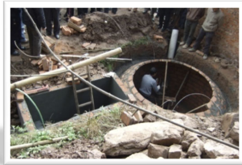
Chamber bricking
