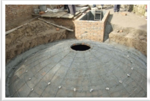
Large chamber buttressing
